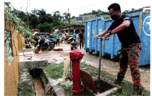
Ng says it costs RM11,000 to replace one underground hydrant with an above-ground pillar hydrant. — Filepic
